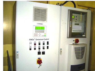
Figure 2-3: SCR Control System
