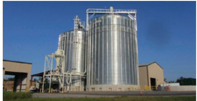
Figure 6.5 | In a project led by TennEra LLC, innovative technologies for (top) handling and (bottom) compacting forage harvester-chopped biomass increased bulk flow rates compared with tub-ground bales, resulting in reduced downstream processing and handling costs.
