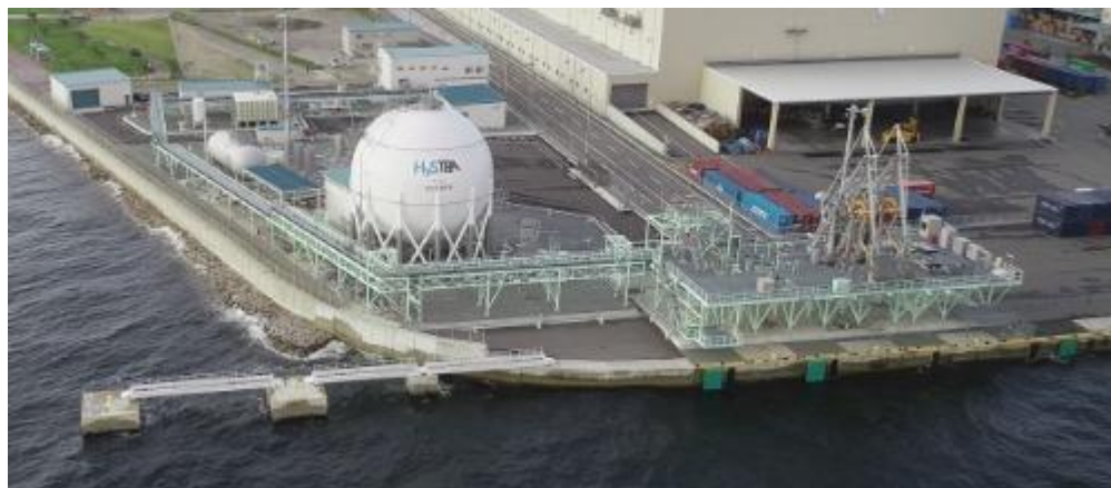
Figure 23: The world's third largest liquid hydrogen tank forms part of an import terminal at Port of Kobe, Japan and can store 178 tonnes 68 (image: HyTouch Kobe).
