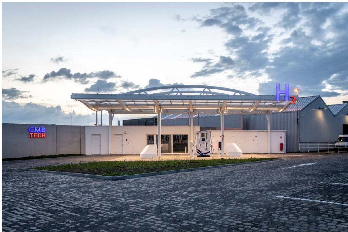
CMB.Tech fixed multi-modal gaseous hydrogen bunkering facility.
